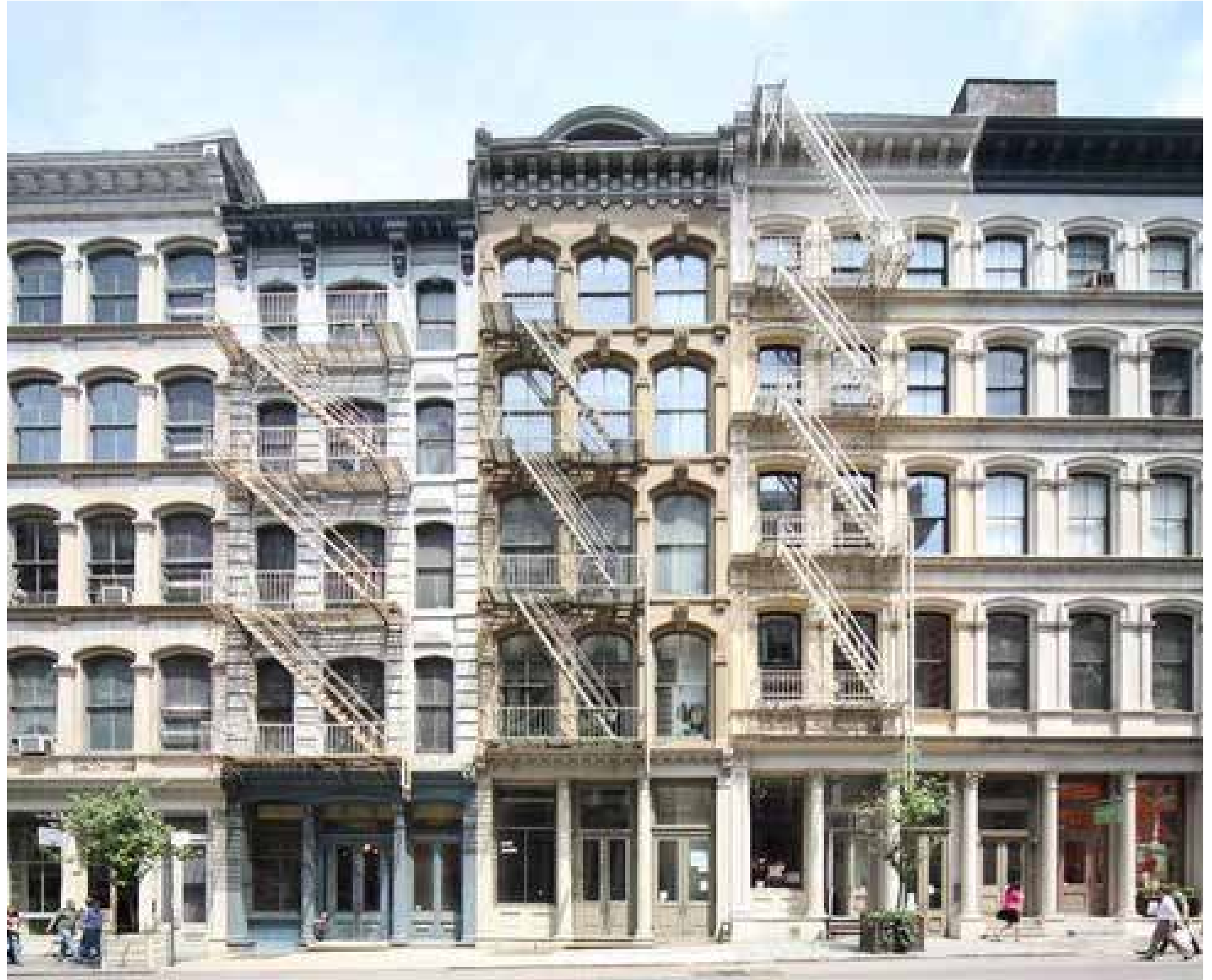
SOHO CAST IRON DISTRICT TYPICAL STREET ELEVATION
