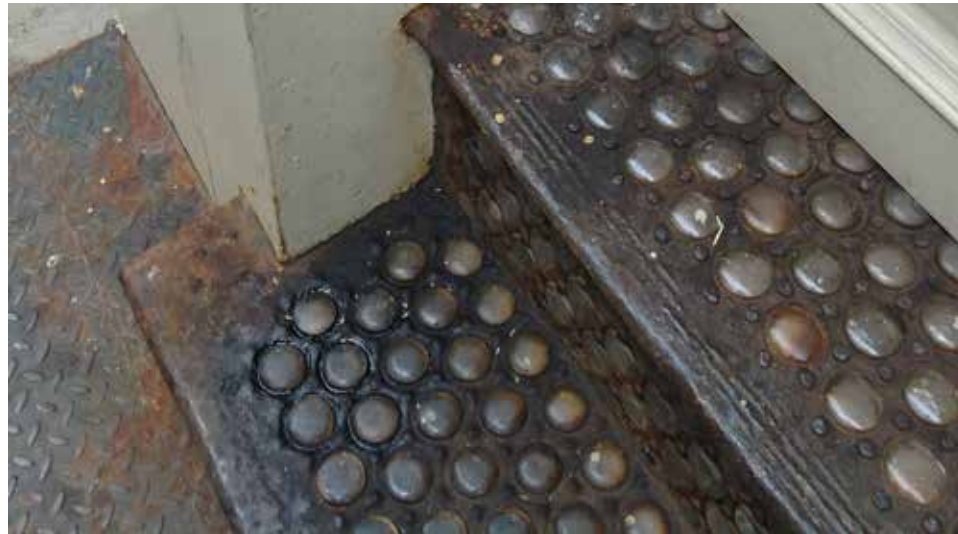
EXISTING SOUTH PRISMATIC VAULT LIGHTS
