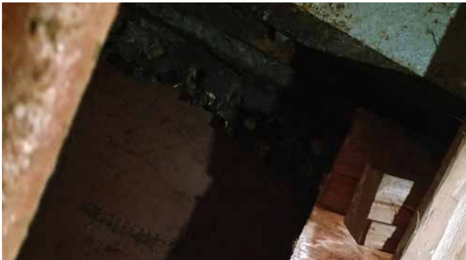
NORTH PRISMATIC VAULT LIGHT CONDITION - DECAY
