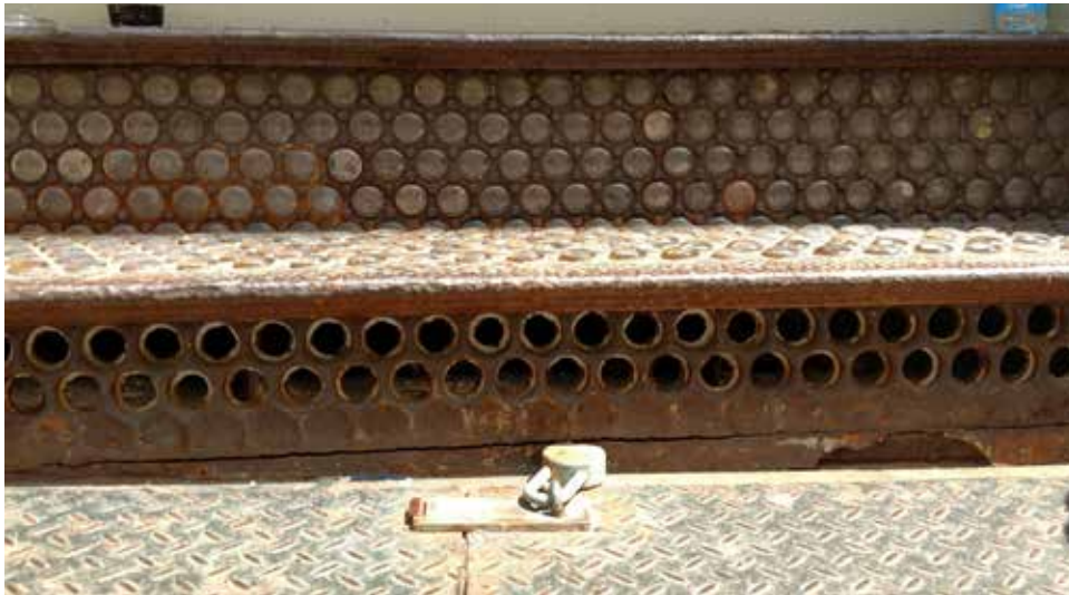
SOUTH PRISMATIC VAULT LIGHT CONDITION
