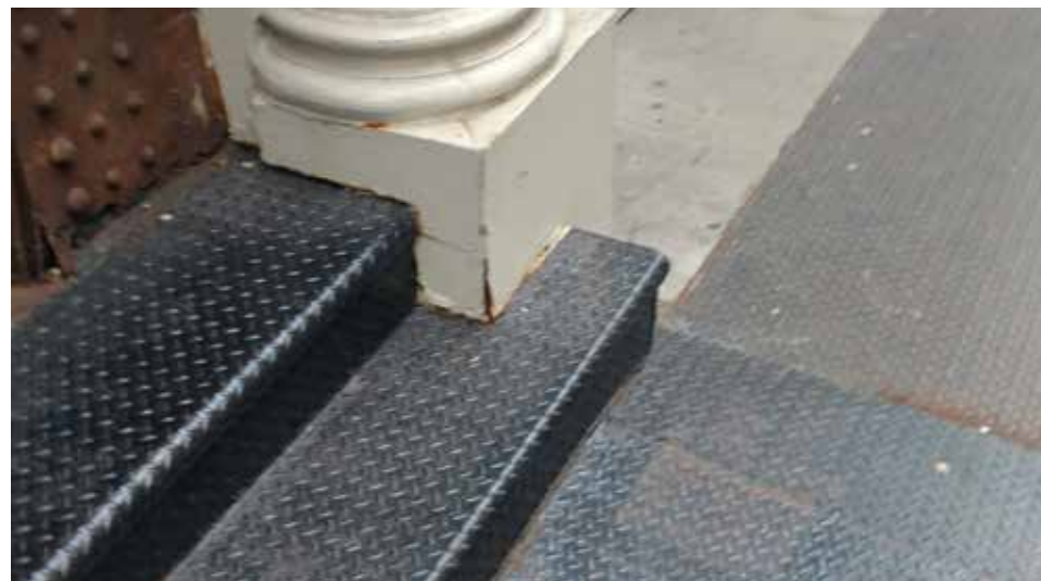
EXISTING DIAMOND PLATE COVERING NORTH VAULT
